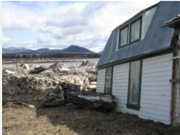
2009 damage to the Eagle Historical Museum from an ice jam on the Yukon
