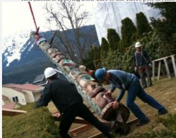
Ron Sheetz is applying Bora-Care to the YaxTe pole in Auke Bay
